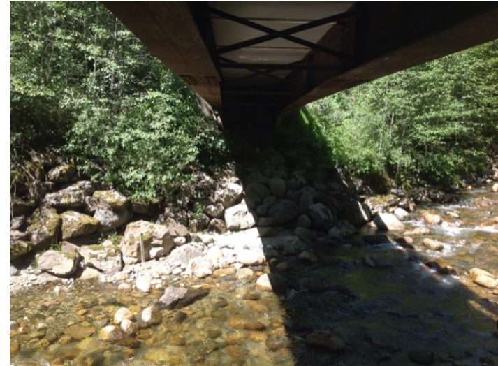
Right Bank Abutment when facing downstream
