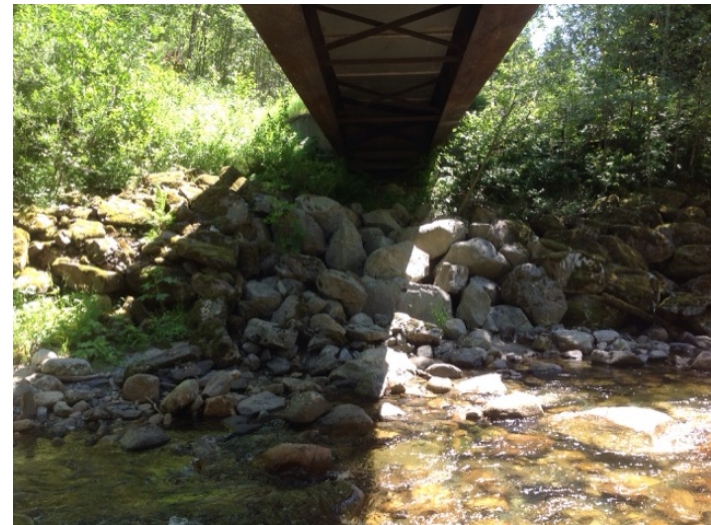
Left Bank Abutment when facing downstream
